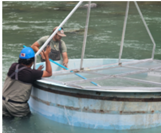
Figure 1 installing a circular tank near the fish fence to reduce impacts to Chinook during holding periods. Photo by Garry John
